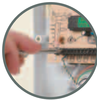
Mounting pulling cable through and wiring the Panel
